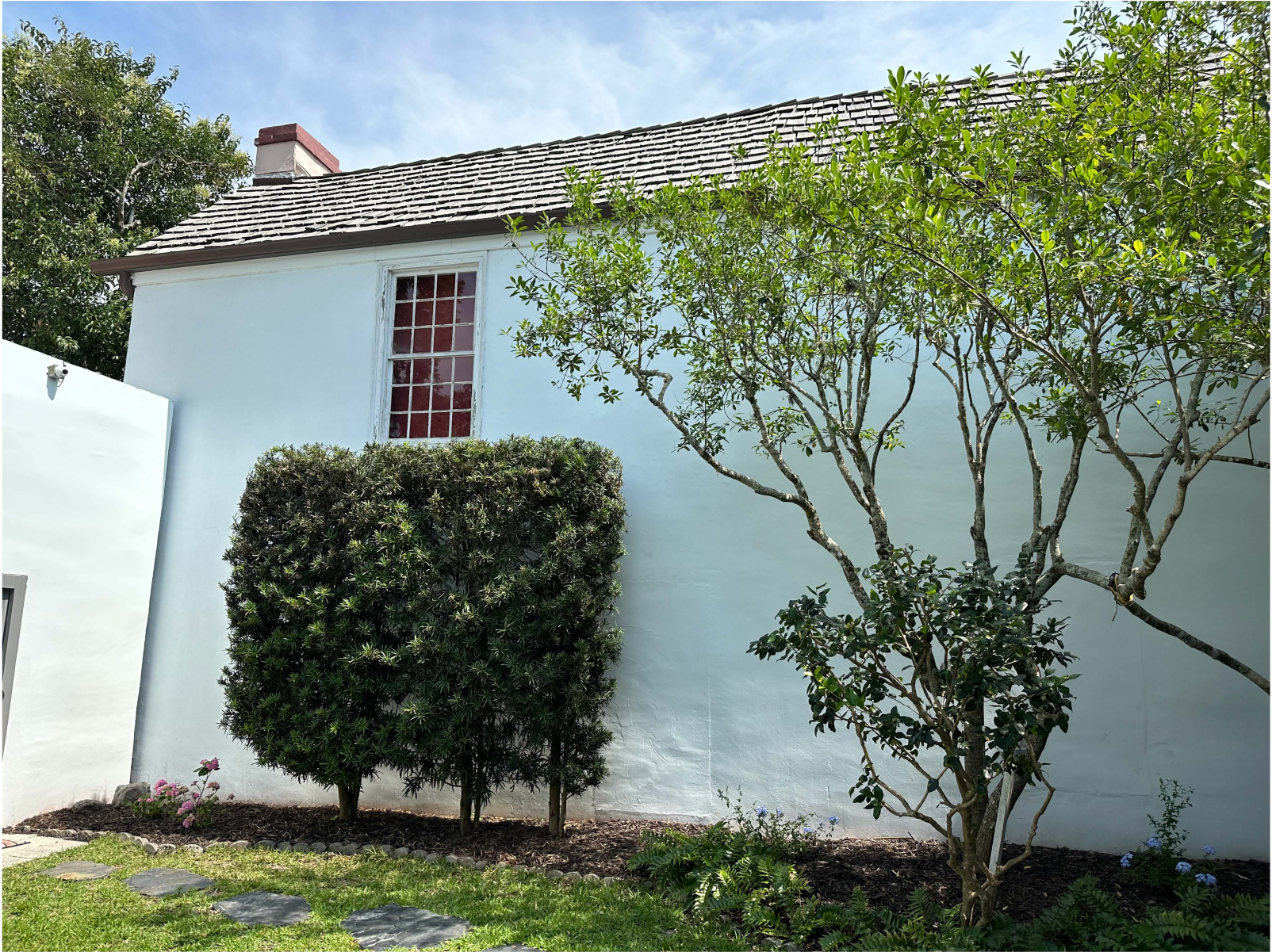
E: East Wing, N facade, looking SE
