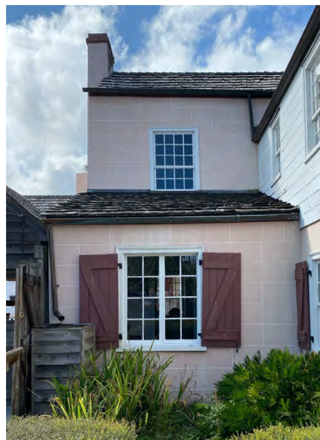
C: West Wing, E facade, looking W and up
