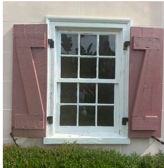
B: East Wing, window 1S2, looking N
