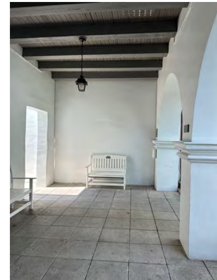
C: East Wing, N facade, looking S.
