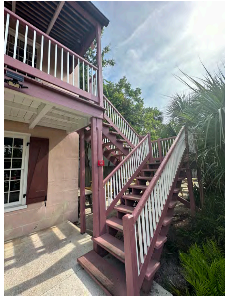
B: East Wing, loggia, looking NE
