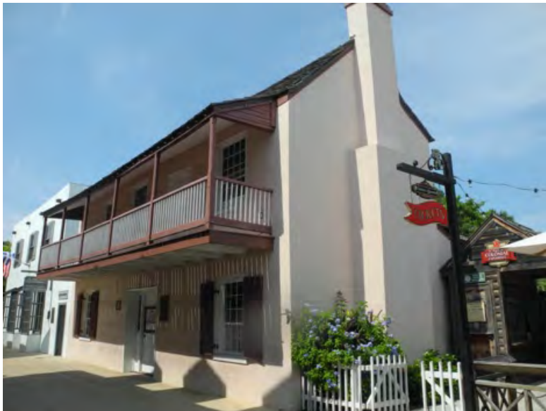
B: West Wing, W and S facades, looking NE
