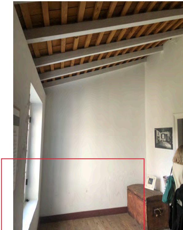
B: Rooms 104 and 105, looking S
