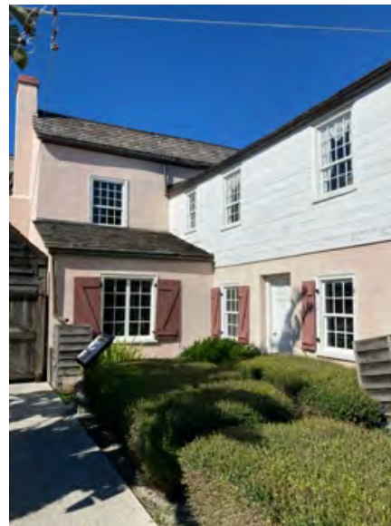
C: East Wing, S facade, looking NW
