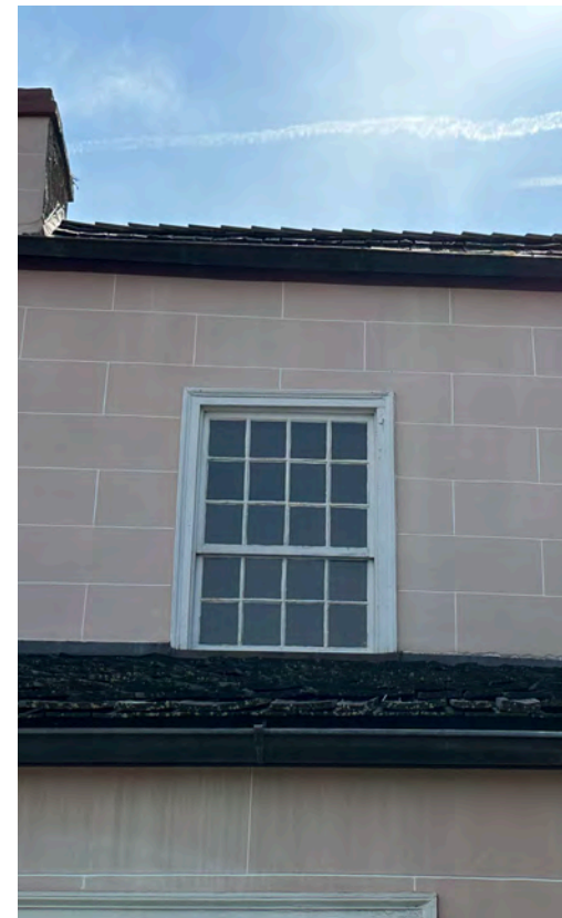
B: West Wing, E facade, window 2E6 looking W
