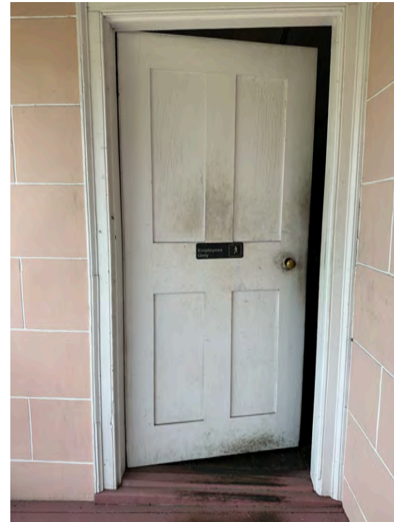
B: Door D24 East Wing, Loggia, looking W
