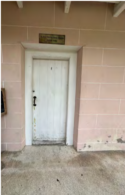
A: Door D11 East Wing, S facade, looking N
