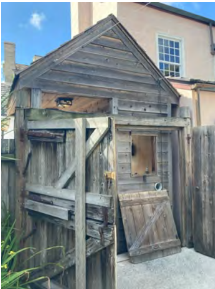
B: Auxiliary structure, looking NE
