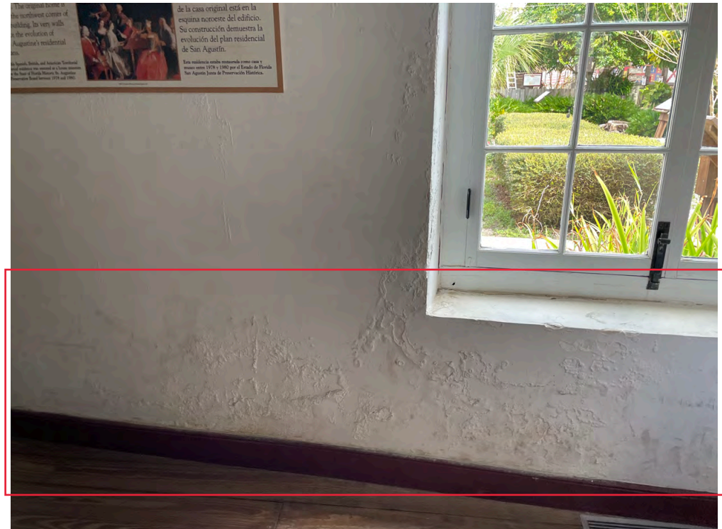
C: Rooms 104 and 105, looking E and down
