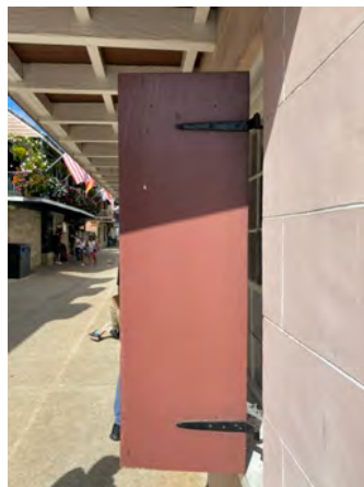
E: West Wing, W facade, looking N
