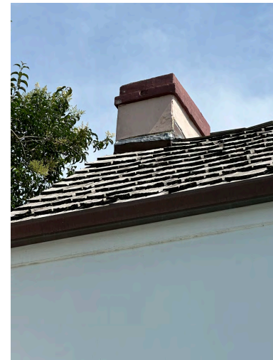
C: East Wing, N facade, looking S
