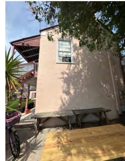
A: East Wing, E facade, looking W
