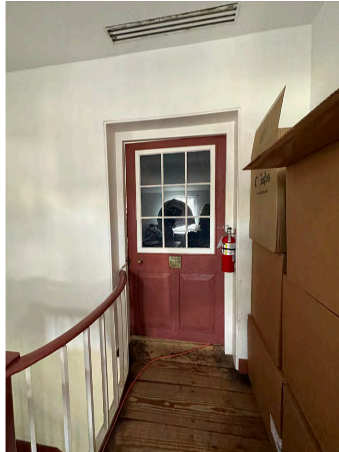
B: Room 204, looking NW
