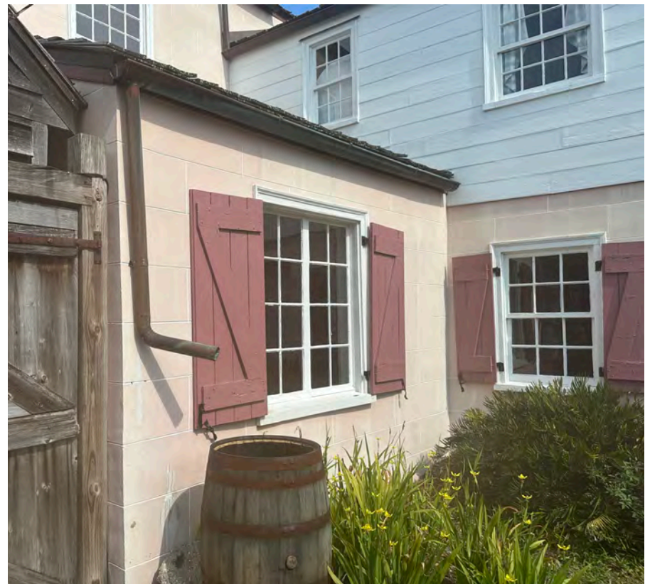
C: West Wing, roof's Eslope, looking NW and up
