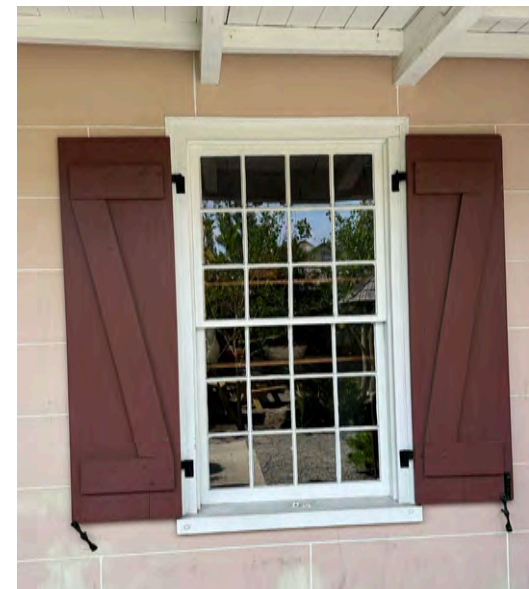
C: East Wing, window 1S1, looking NE
