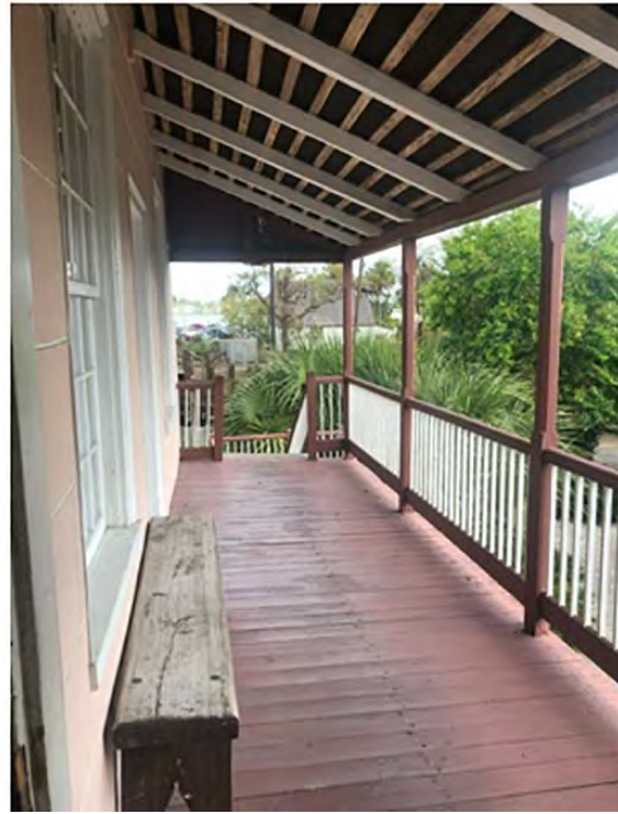
B: East Wing, Loggia, looking E
