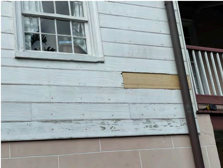
C: East Wing, S facade, looking NE, November 2022
