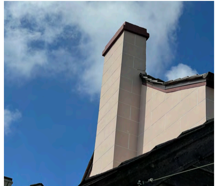
C: West Wing, W wall chimney, looking NW and up
