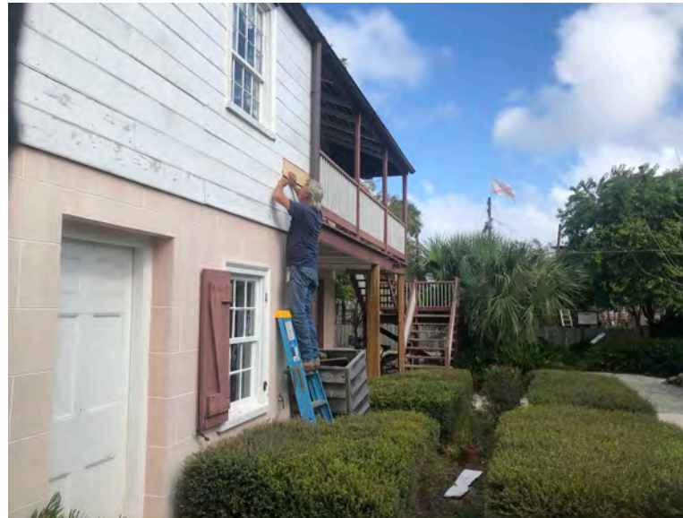
C: East Wing, S facade looking E
