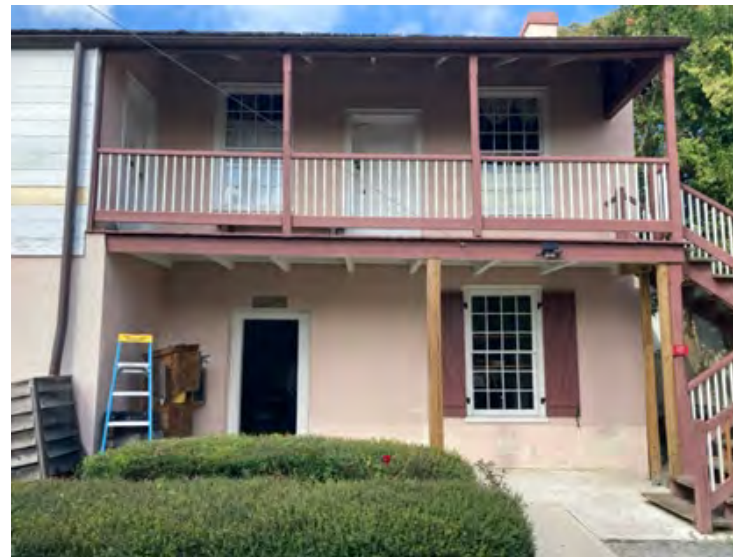
B: East Wing, S facade, looking N
