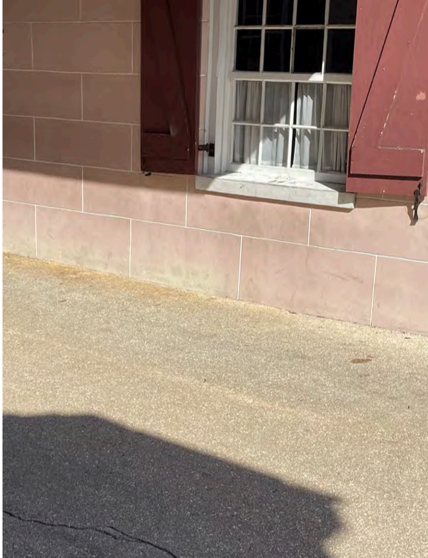
A: West Wing, W facade, looking NE
