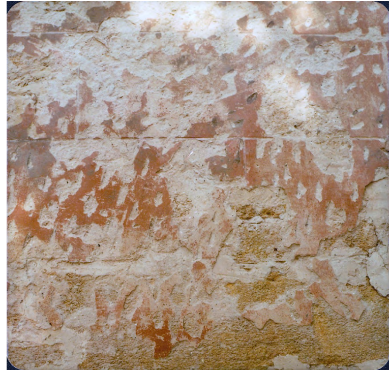
Figure 2 Stucco on East Façade of DeMesa-Sanchez House, 1979. https://ufdc.ufl.edu/USACH00421/00020/citation
