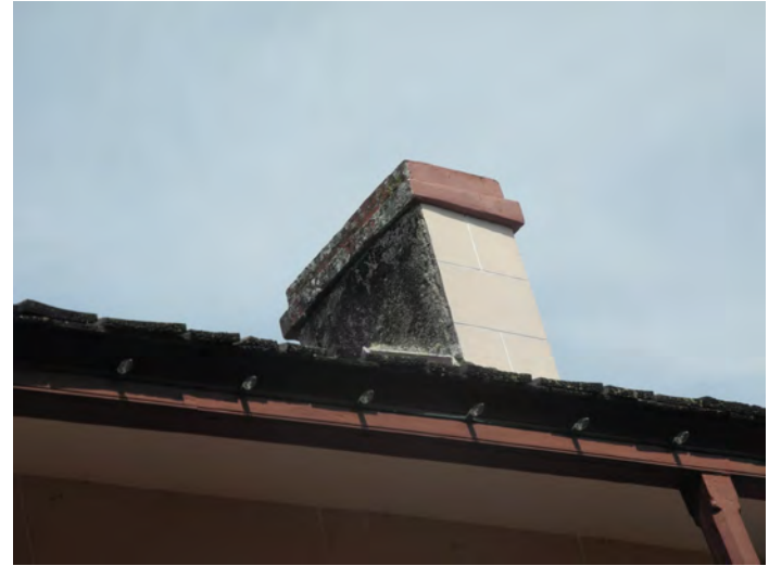
B: West Wing, W wall chimney, looking SE and up
