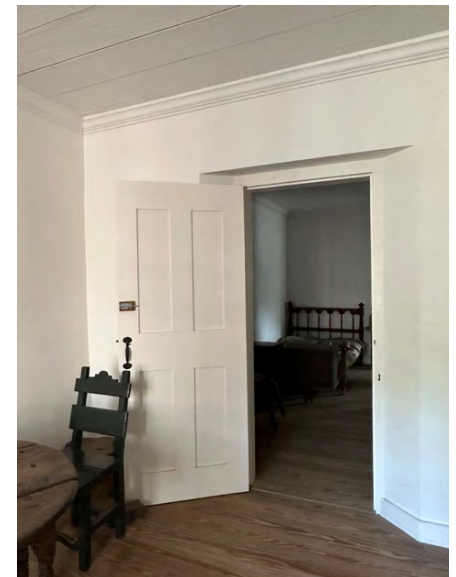
D: Room 103, looking NE, door D5
