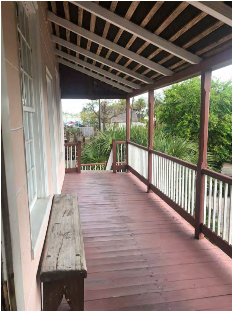
A: East Wing, loggia, looking E
