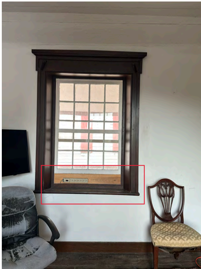
A: Room 201, looking W
