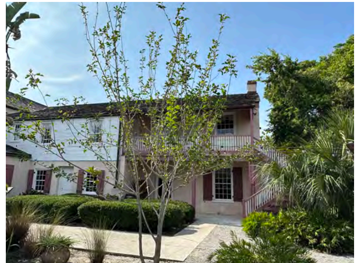
E: Concrete walkway, looking NW
