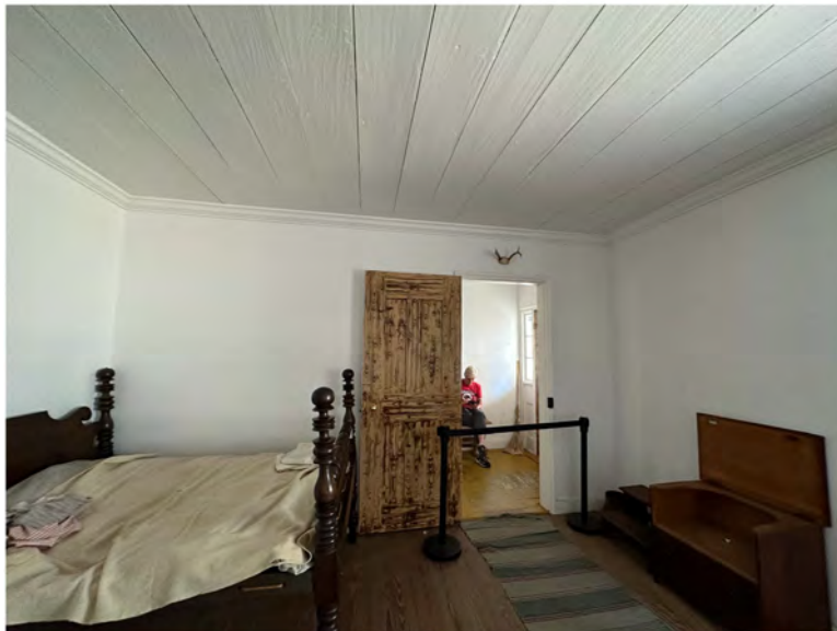
C: Room 103, looking SW
