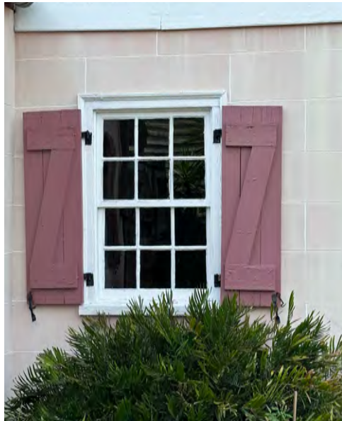
A: East Wing, window 1S3, looking N
