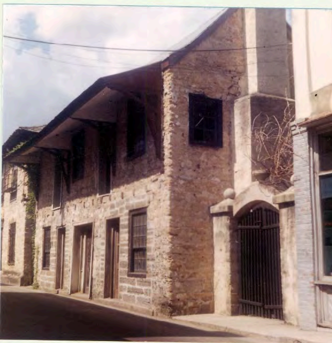
Figure 8 West Wing, west façade, prior to restoration of the balcony, looking Northeast, ca. 1958. https://original-ufdc.uflib.ufl.edu/USACH00551/00080/1x
