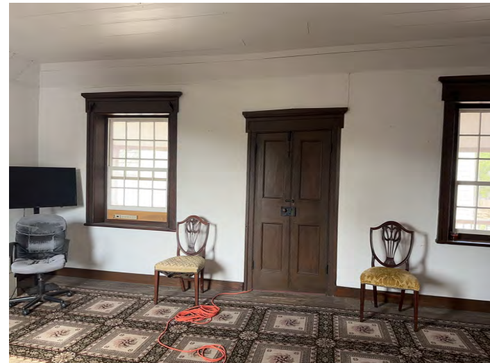
B: Room 201, W wall, looking SW
