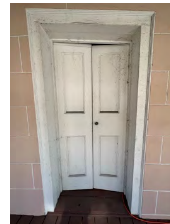
G: West Wing, W facade, looking E
