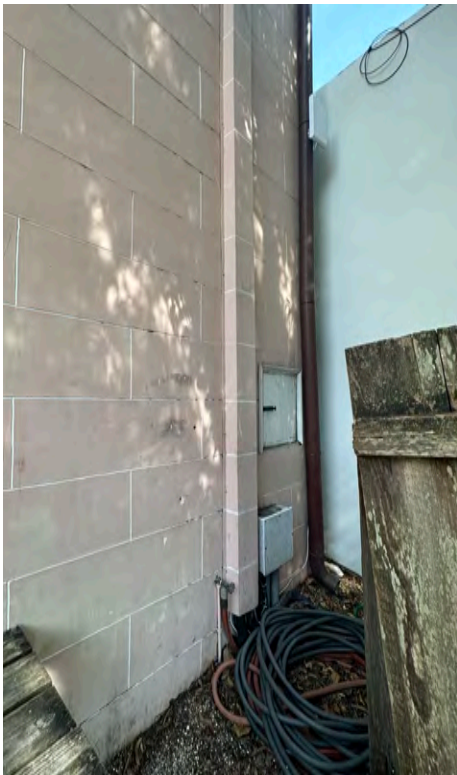
A: East Wing, east facade, looking NW
