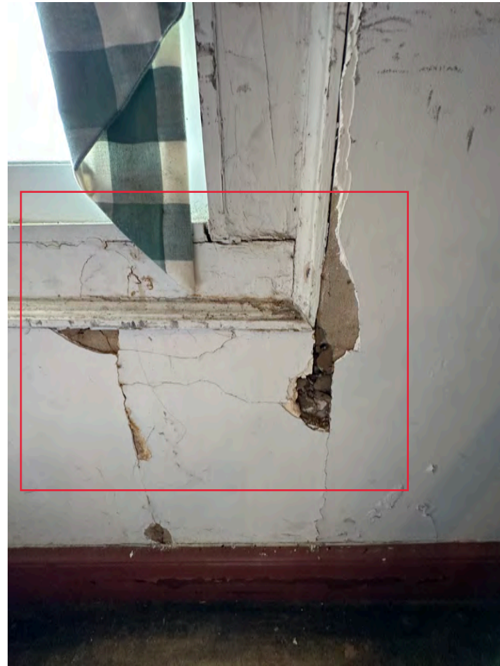
B: Room 207, looking S
