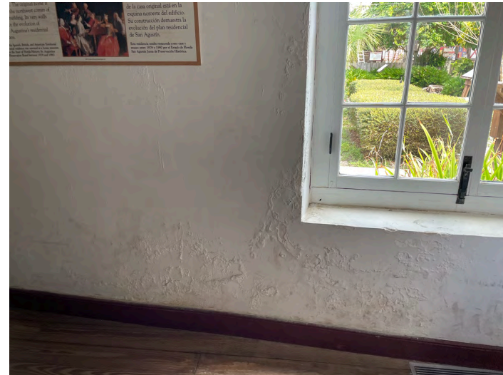
A: Room 104, E wall, looking SE and down
