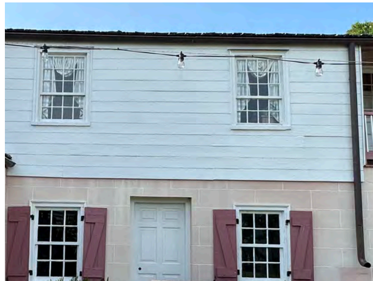
D: East Wing, S facade, looking N, June 2022
