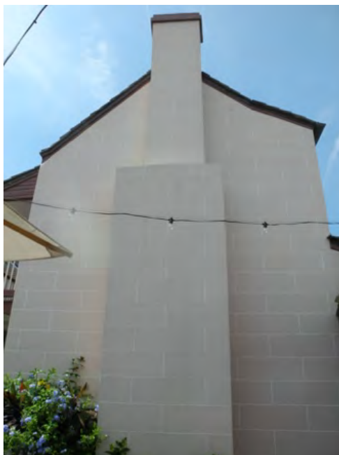
A: West Wing, S facade, looking N and up
