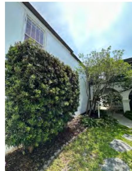
D: East Wing, N facade, looking E
