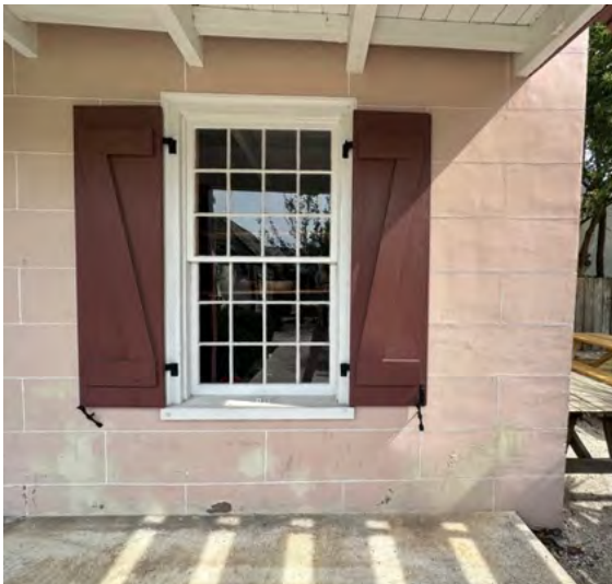
D: East Wing, Loggia, looking N
