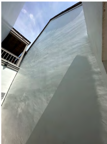
A: West Wing, N facade, looking SE and up.
