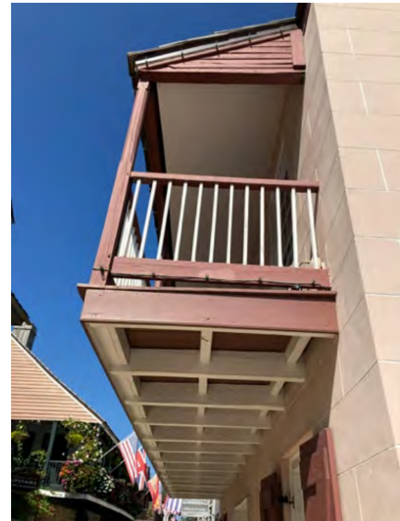
B: West Wing, balcony, looking N and up
