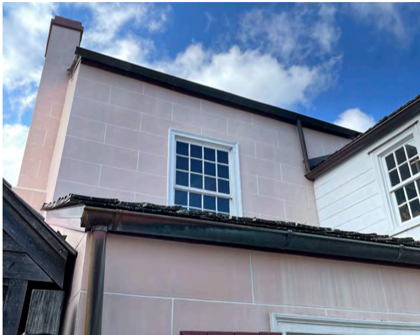
B: West Wing, E facade, looking NW
