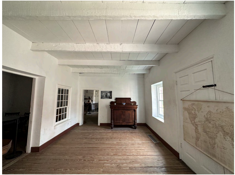
B: Room 107, looking E
