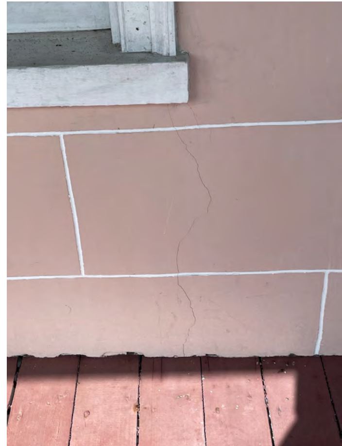
C: East Wing, S facade, looking N
