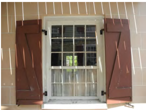
D: West Wing, W facade, looking E
