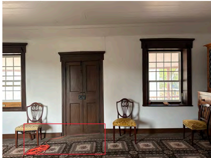
A: Room 201, looking W
