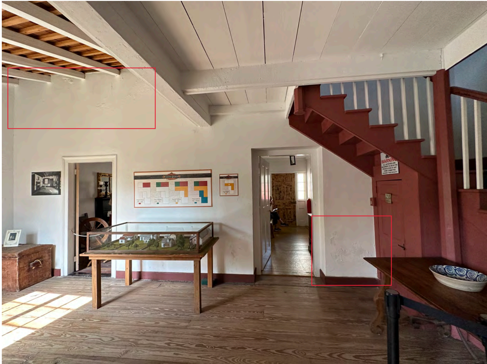
A: Rooms 104 and 105, looking SW
