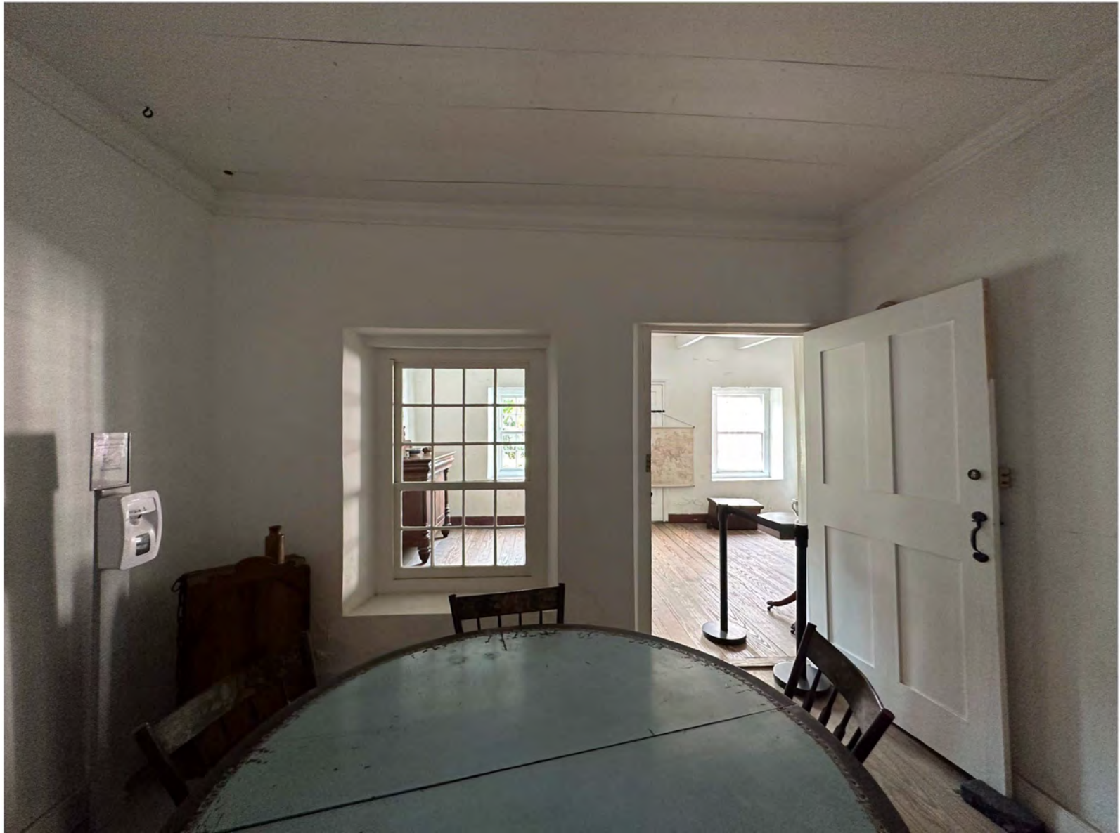
A: Room 108, looking S
