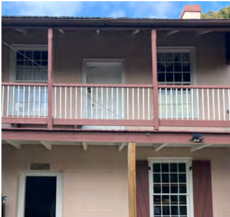
A: Door D23 East Wing, S facade, looking N
