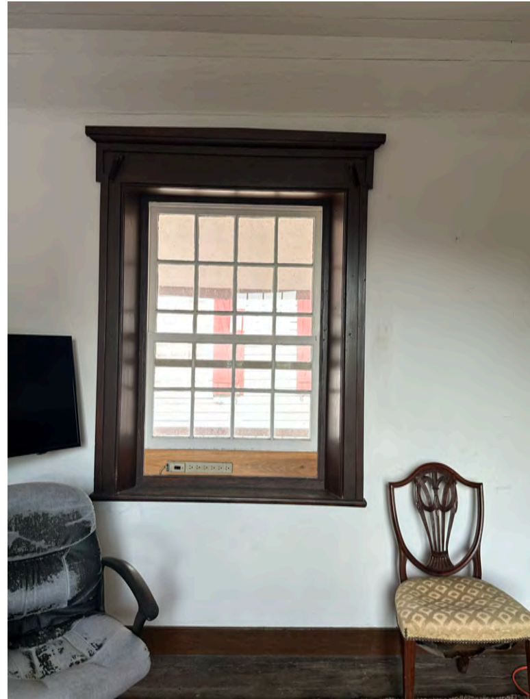
B: Window 2W1, looking W
