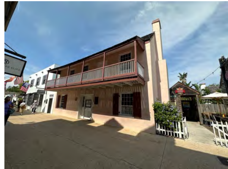
A: West Wing, W facade looking NE
