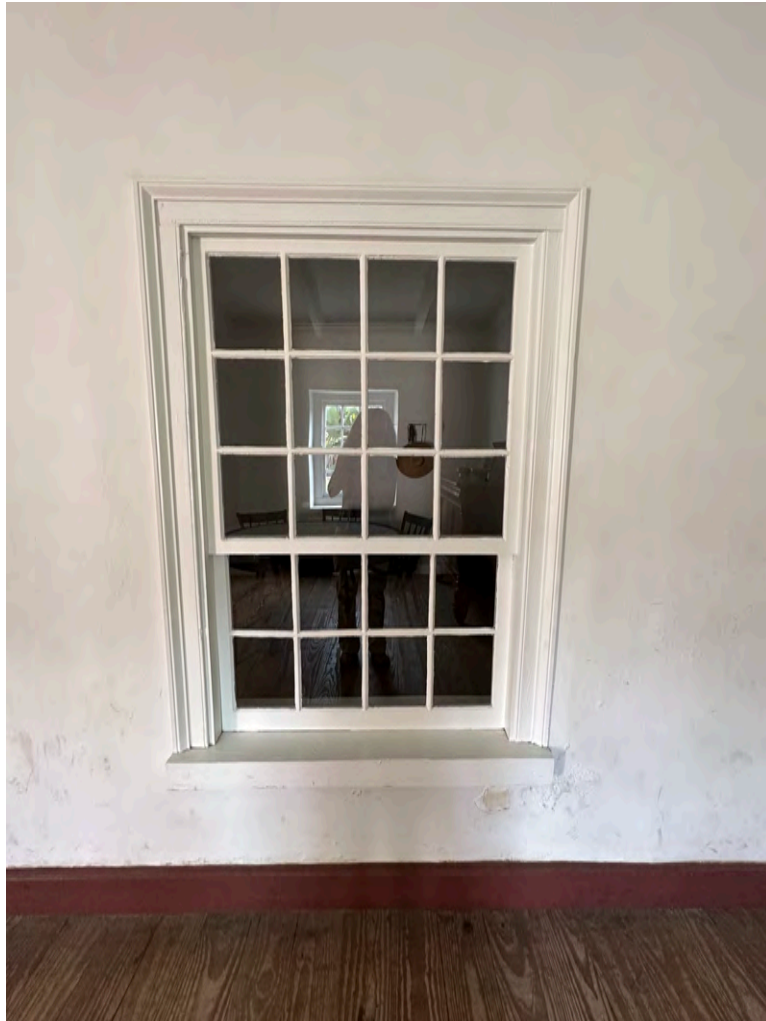
A: Window 111, looking N
