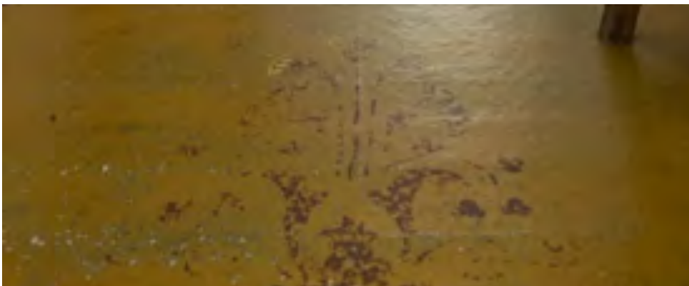
C: Room 102, looking E and down
