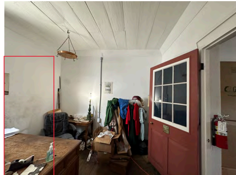
B: Room 206, looking E
