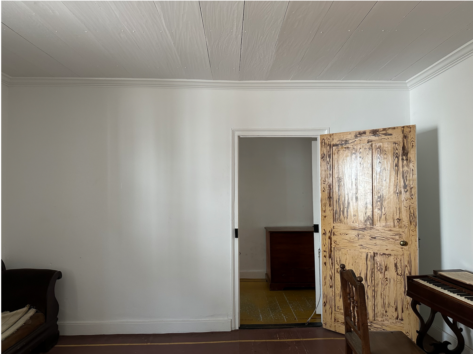
C: Door 2D, looking N
