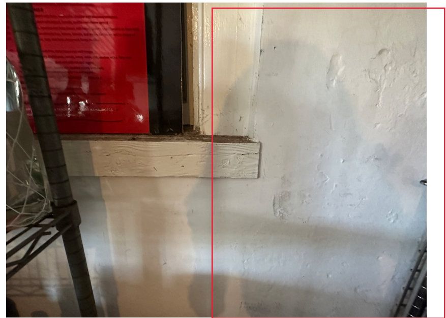
B: Room 210, window 2N1, looking N
