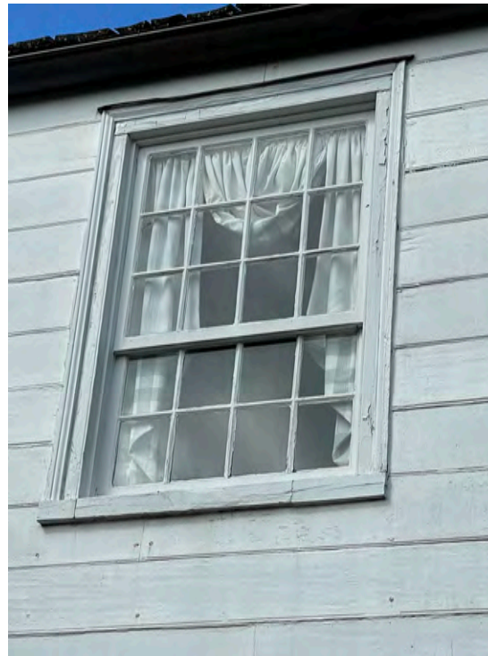
B: East Wing, window 2S4 looking NE and up
