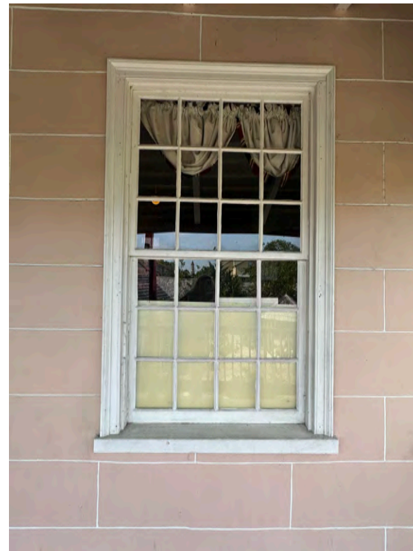
B: East Wing, window 2S1, looking N
