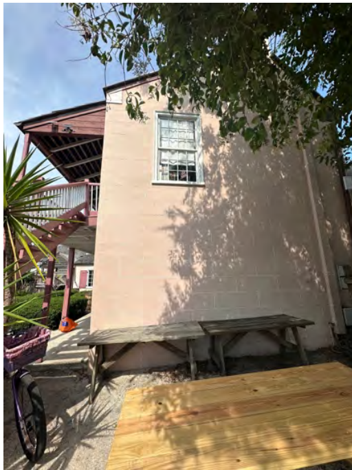
A: East Wing, S facade, looking NW
