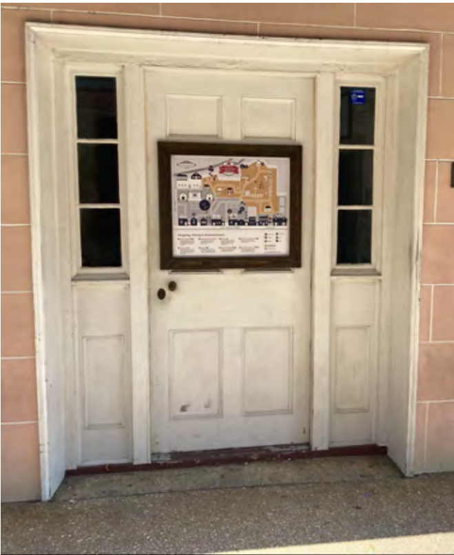
A: Door D1 West Wing, W facade, looking E
