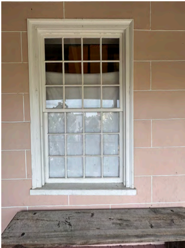
A: East Wing, window 2S2, looking N
