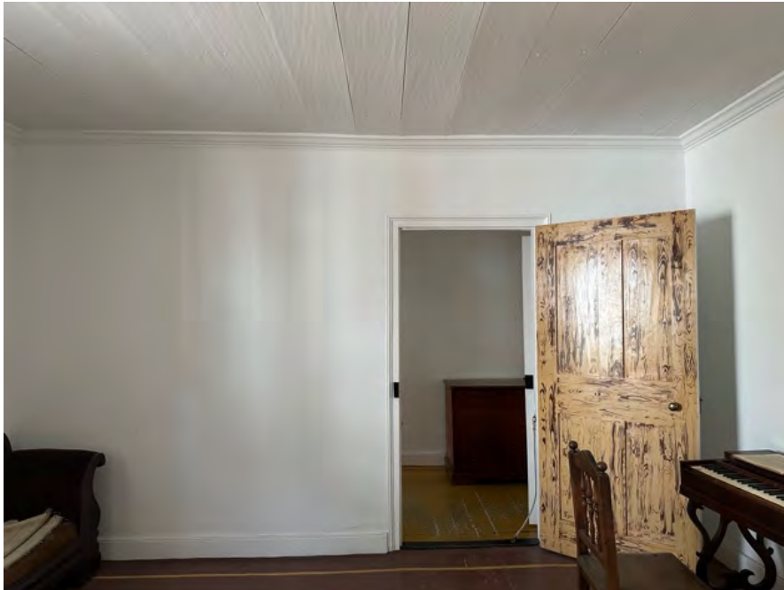
B: Room 101, looking N
