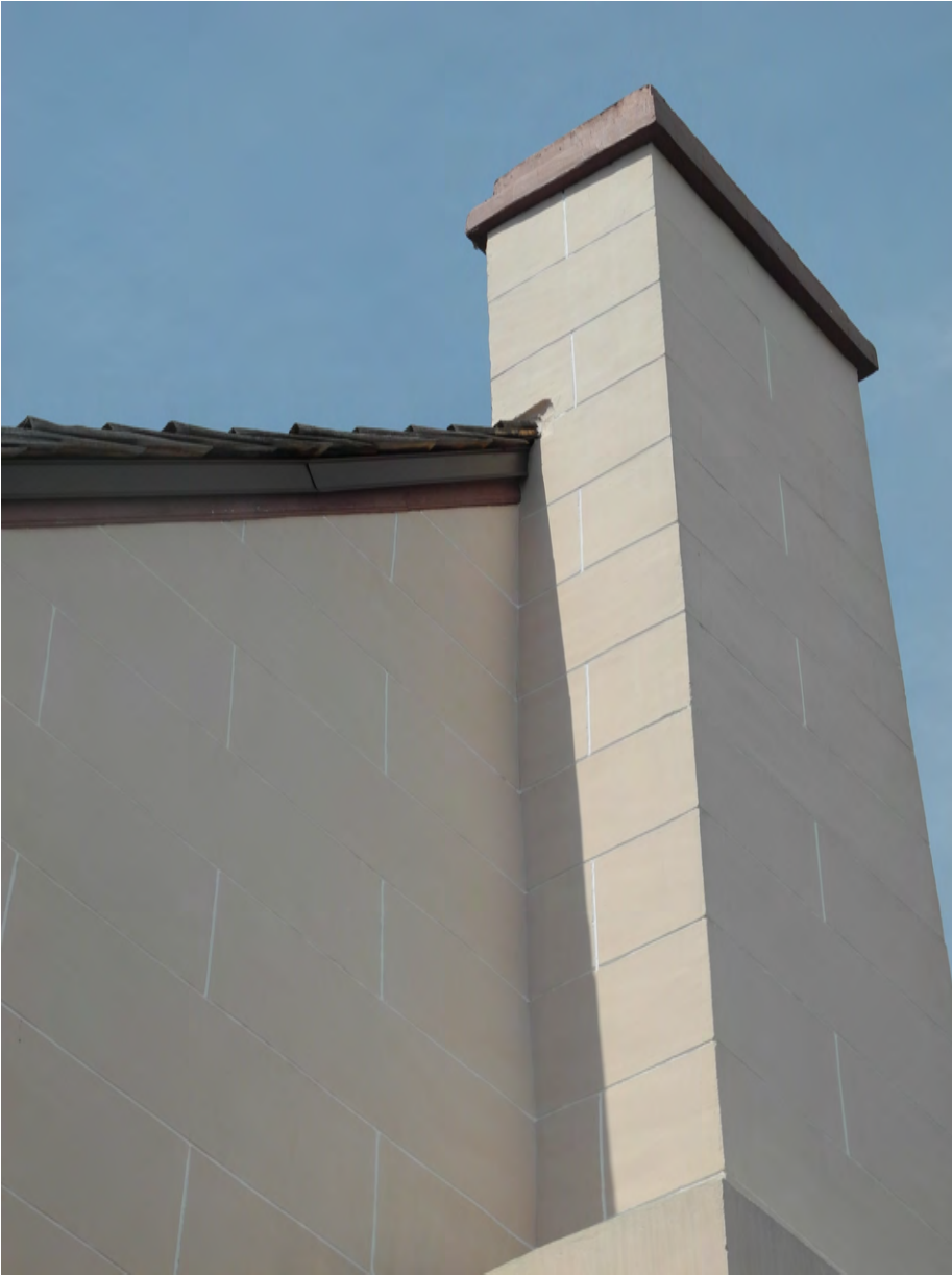
A: West Wing, W wall chimney, looking NE and up
