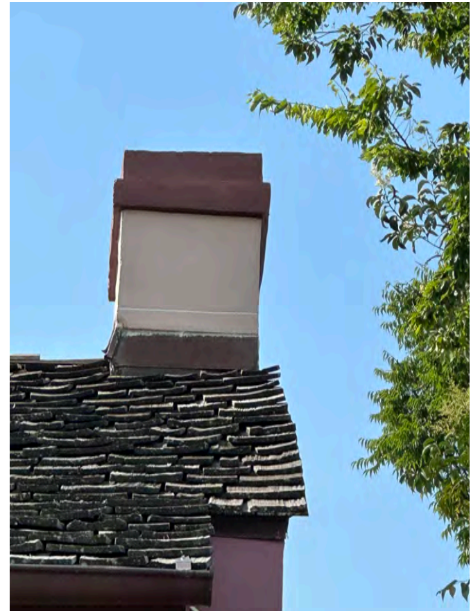
E: East Wing, E wall chimney, looking N and up
