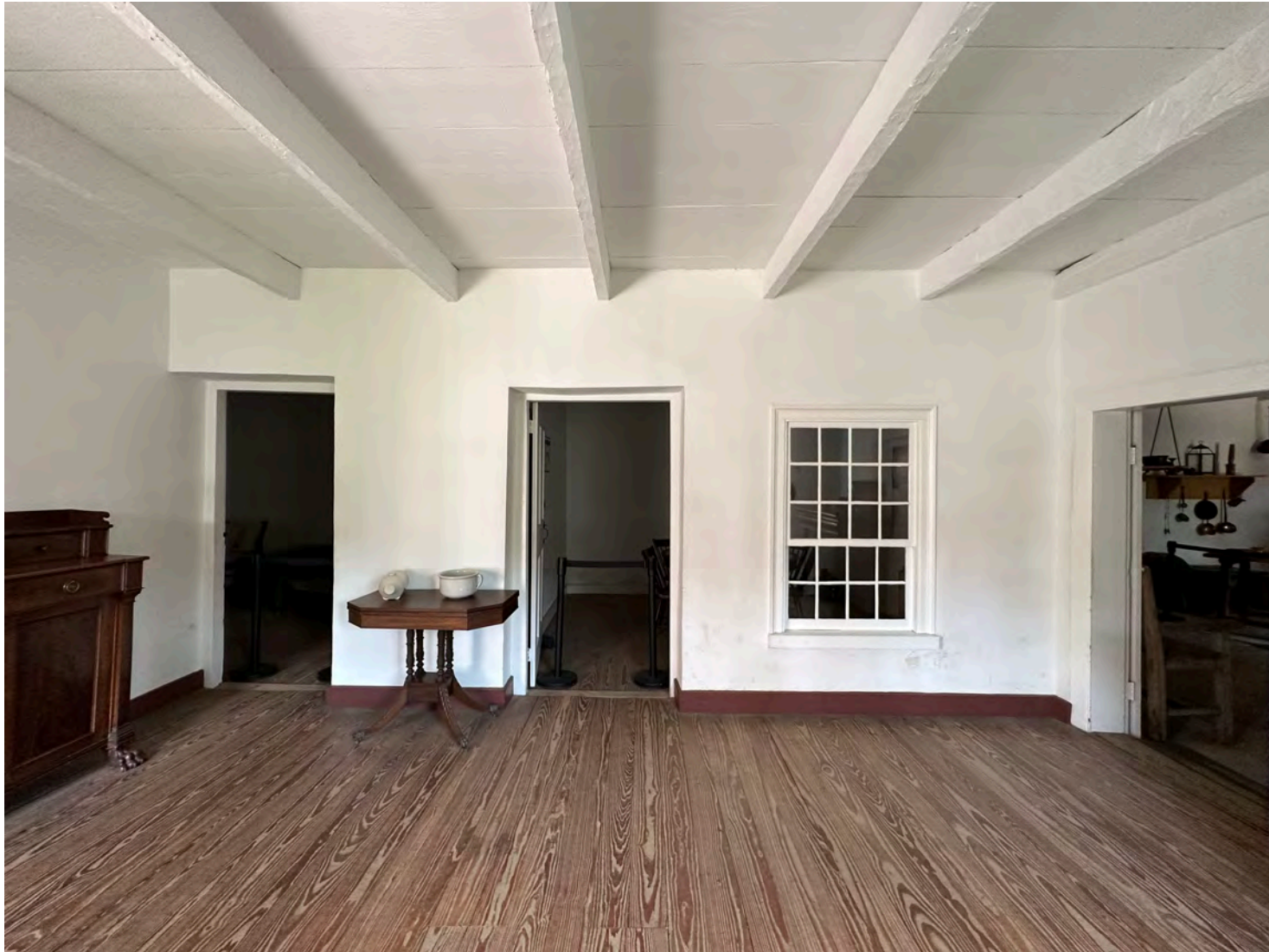
A: Room 107 looking N
