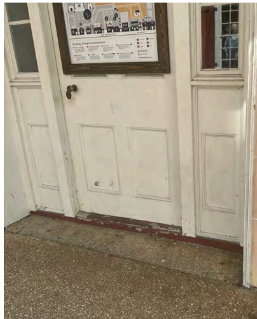
B: Door D1 West Wing, W facade, looking NE
