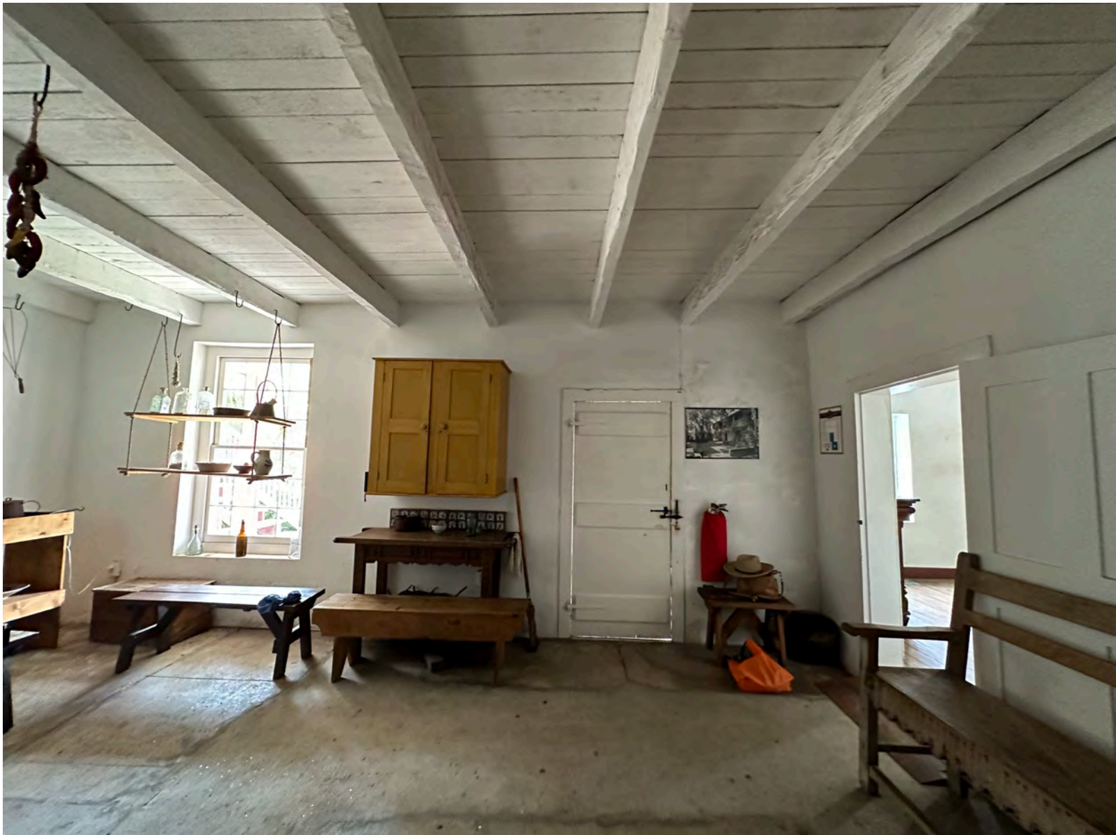
A: Room 110, looking S
