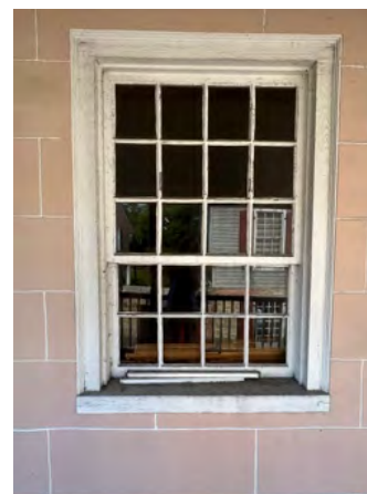
F: West Wing, W facade, looking E
