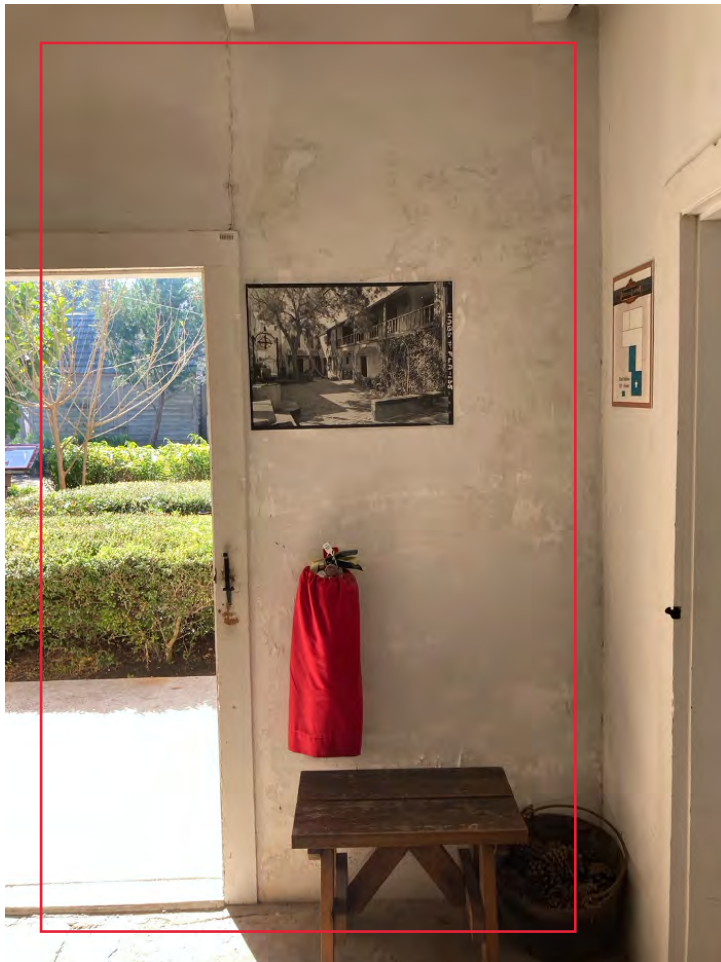
A: Room 110 , looking S
