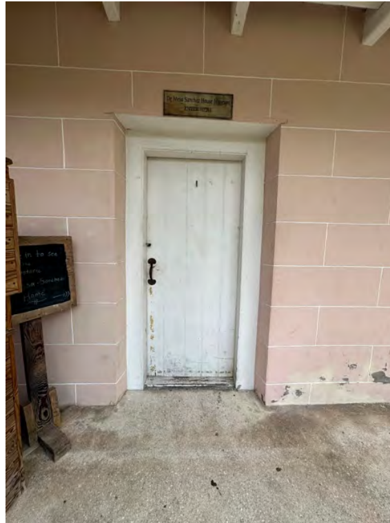
C: East Wing, S facade, door D11
